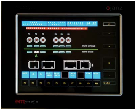
Figure 3: Tram diagnostic screen
